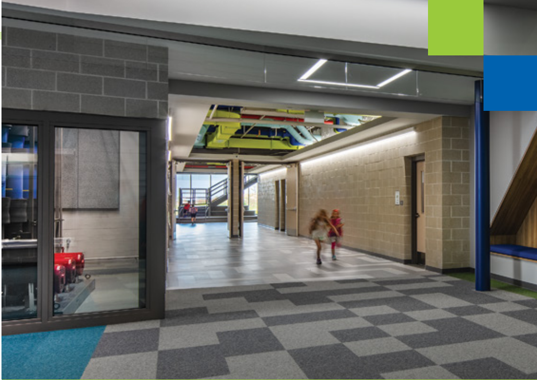
A part of the ceiling at Token Springs Elementary School has been removed to reveal pipes that students can trace into the adjacent geothermal pump room.
